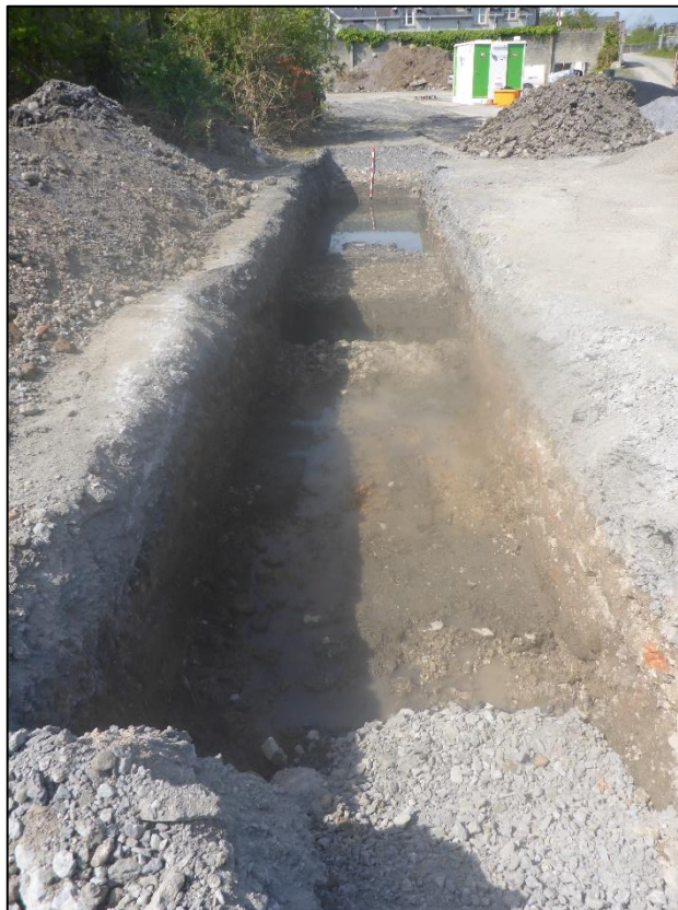
Plate 8. Overview of Test Trench 7, facing north.
