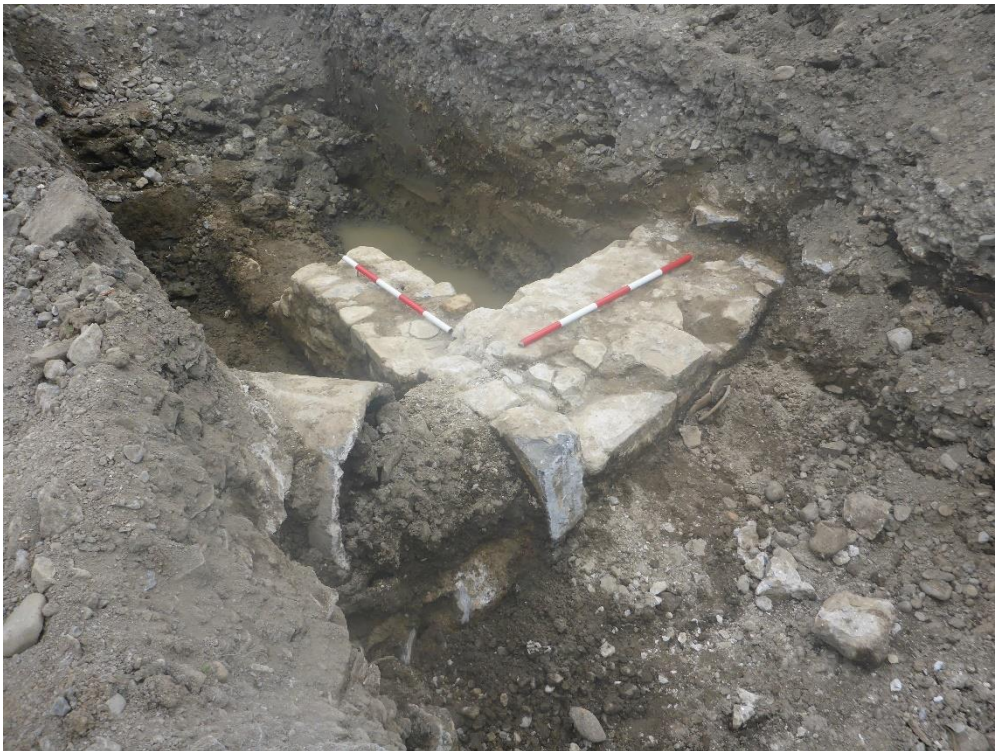
Plate 16. Disturbance to wall in Test Trench 11 from modern concrete pipe, facing northwest.
