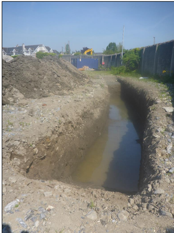
Plate 10. Overview of Test Trench 8, facing north.
